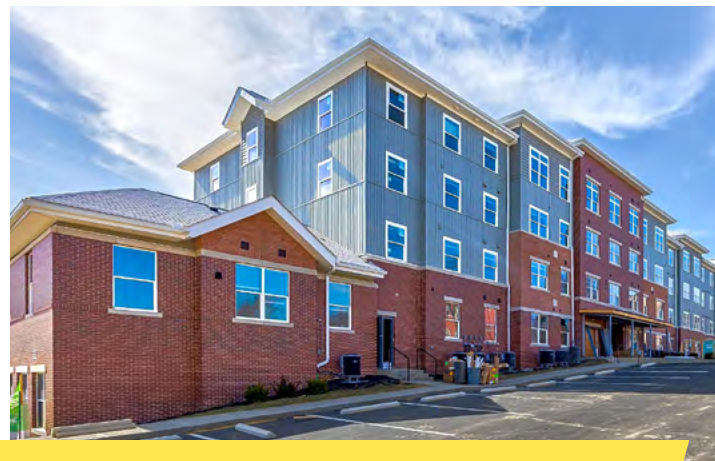
Blair Lofts is a new affordable housing complex in Avondale.
