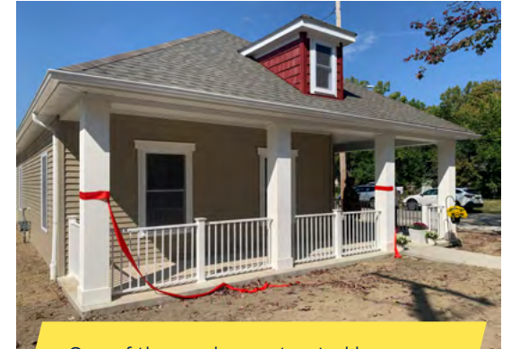
One of the newly constructed homes that is part of the Larchmere Homes 30 affordable lease-to-purchase homes in the Buckeye Neighborhood.
