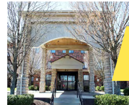
Hoover Place has 144 units of affordable senior housing for Dayton residents.
